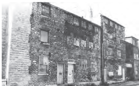
Typical workshops in Sheffield
